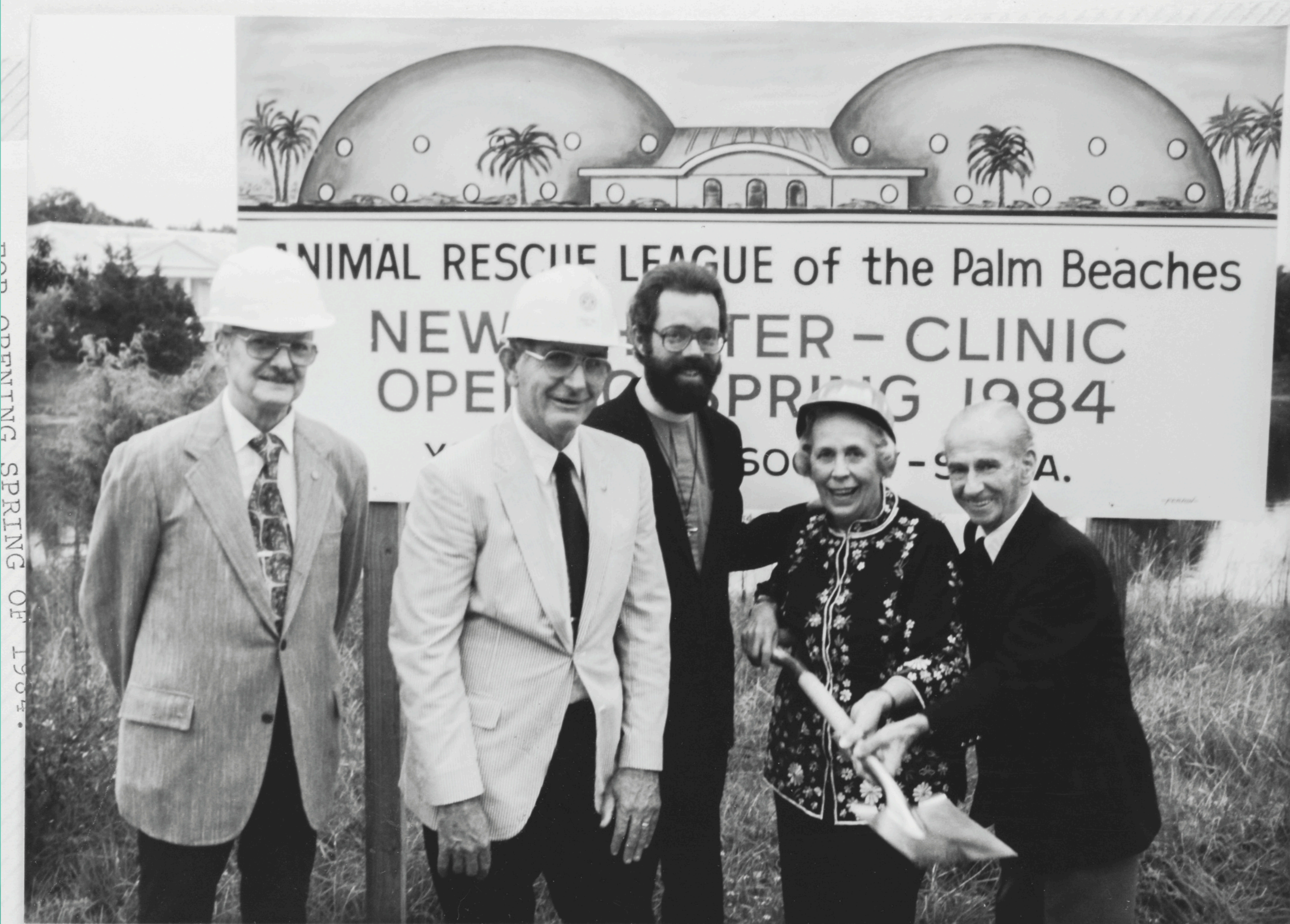
GROUND BREAKING FOR NEW ANIMAL RESCUE LEAGUE SHELTER AND CLINIC
